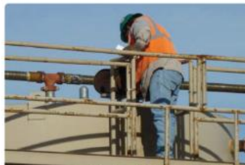
A worker collecting a sample from the open hatch of a production tank. Image: J.D. Damri, OSHA.
